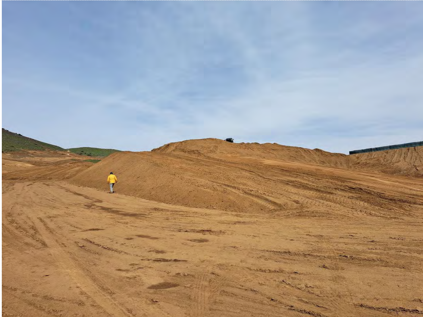
Stockpile of +/- 120,000 cubic yards of dirt
