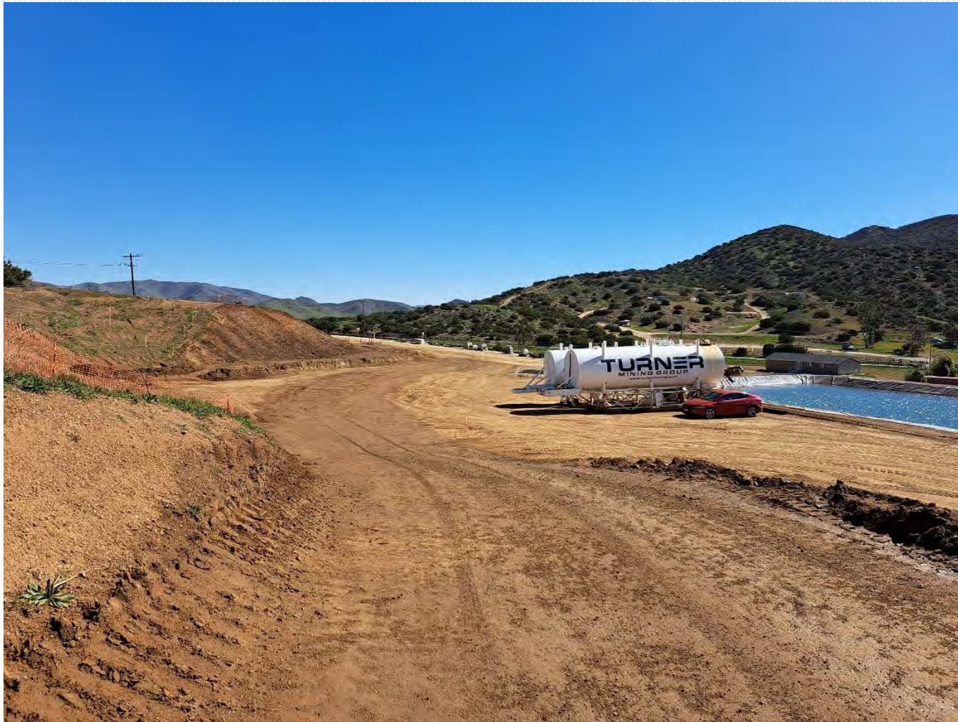
Picture showing completed grade at the Valley Sage Road entrance.
