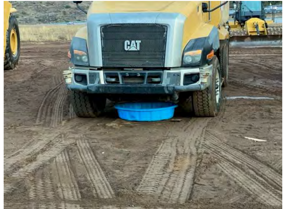
Drip pans for spill prevention and control ( BMP WM-4 )
