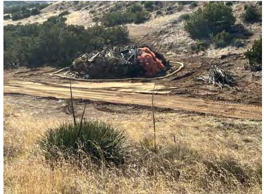
Waddles installed around junk pile
