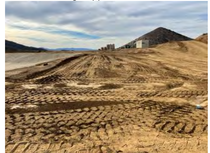
3. Preparation for water truck loading area
