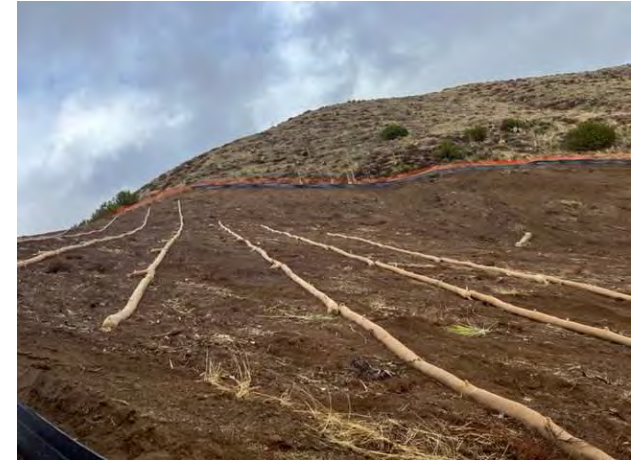
Straw waddle installation see Fig 1
