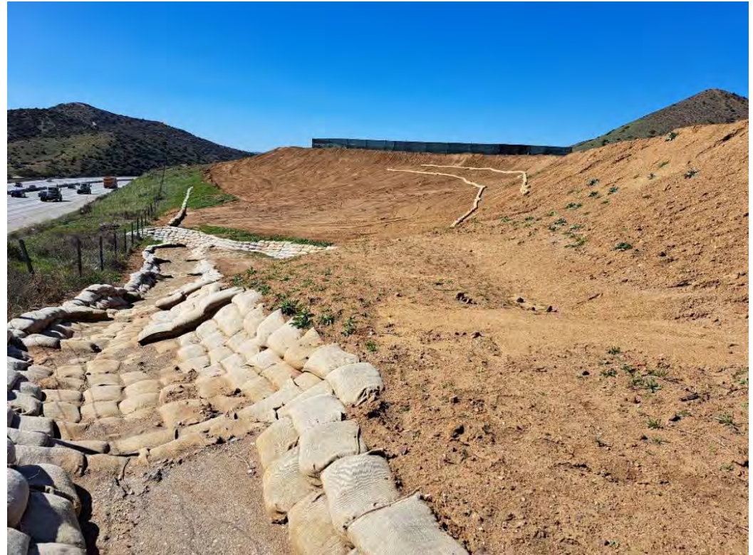
SWPPP installed using wattles and sandbags along highway 14 below the pond and construction equipment pad which are closest to the freeway.
