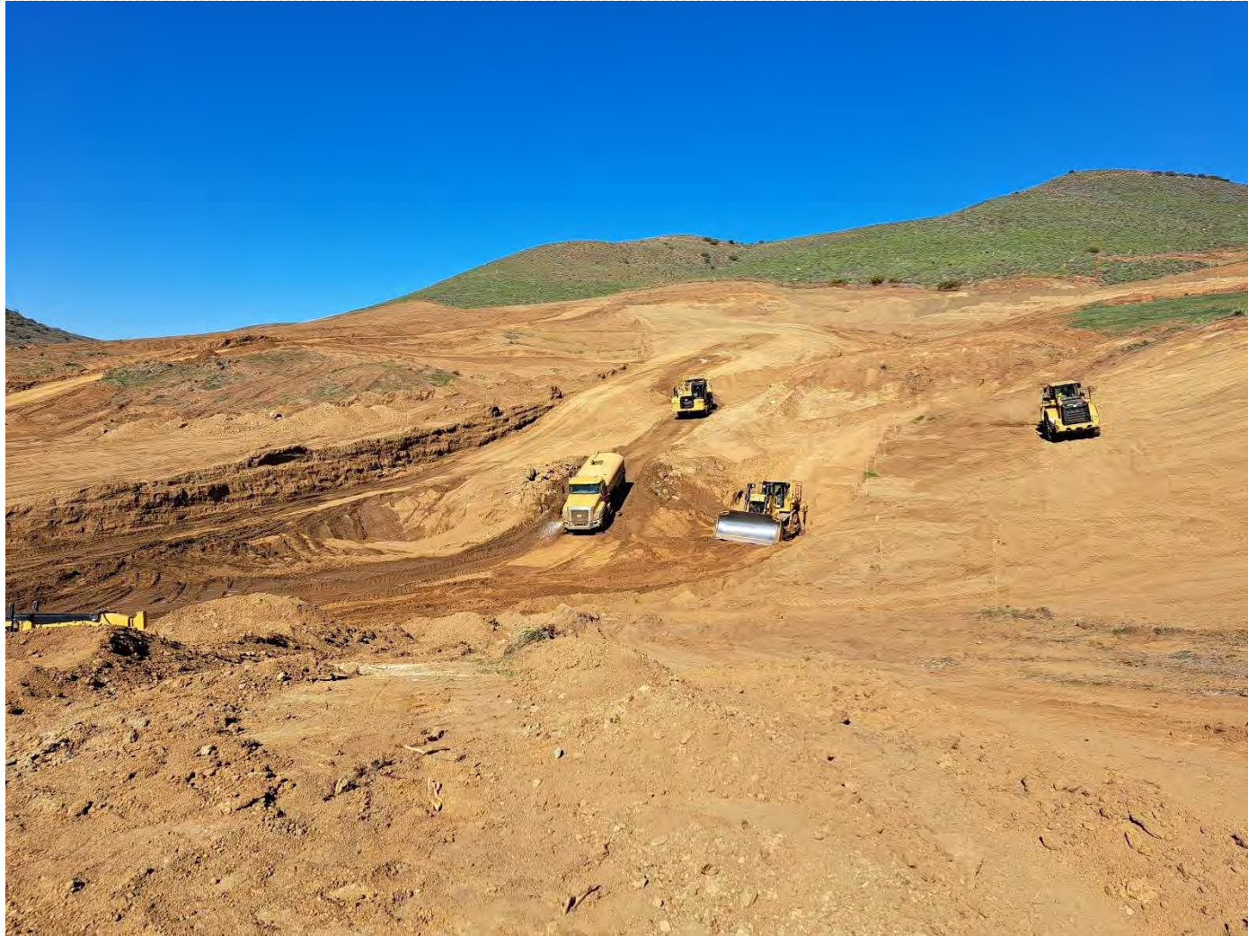
Verification of bedrock as per the RMA Geoscience specification and requirements.
