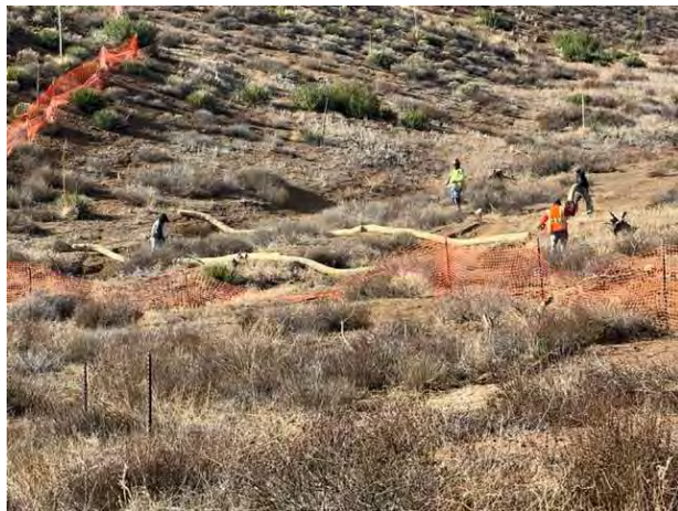
waddles installed in lower riparian areas. see Fig 1
