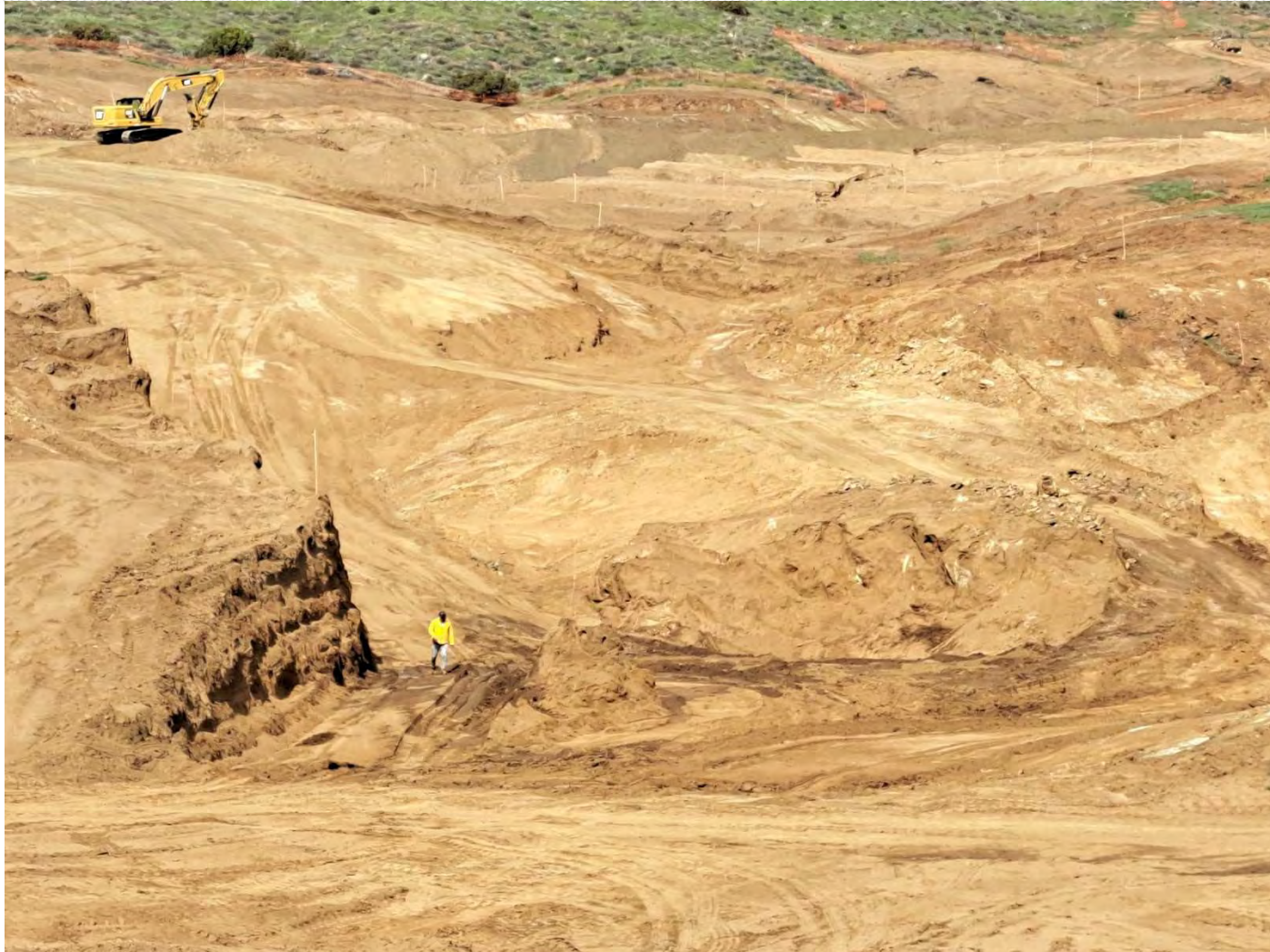
Picture showing exposed bedrock. (Dug up to 30-40 ft down)
