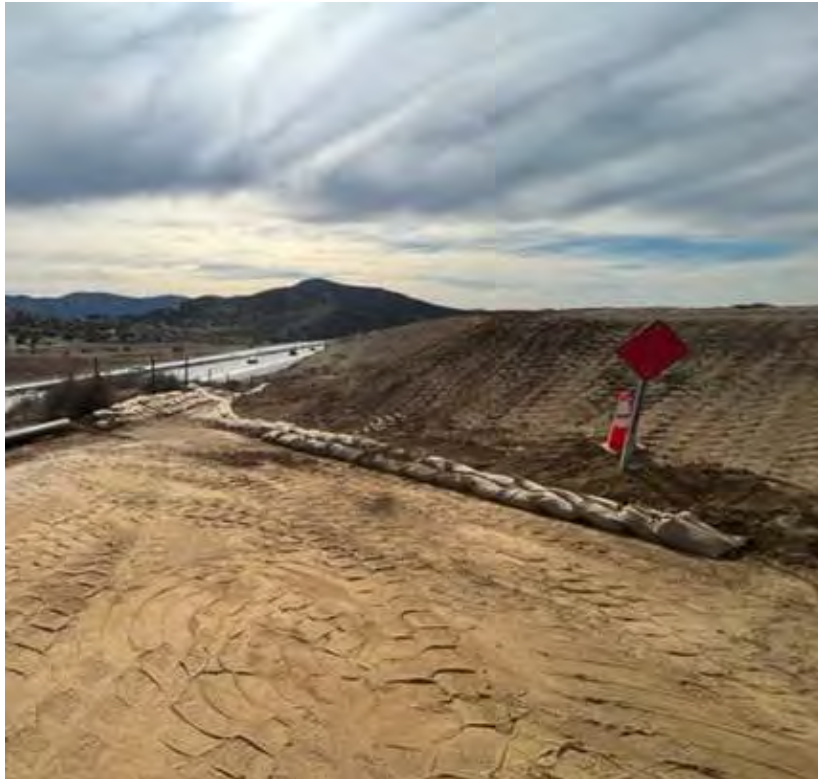
SWPPP installed using wattles and sandbags along highway 14 below the pond and construction equipment pad which are closest to the freeway.
