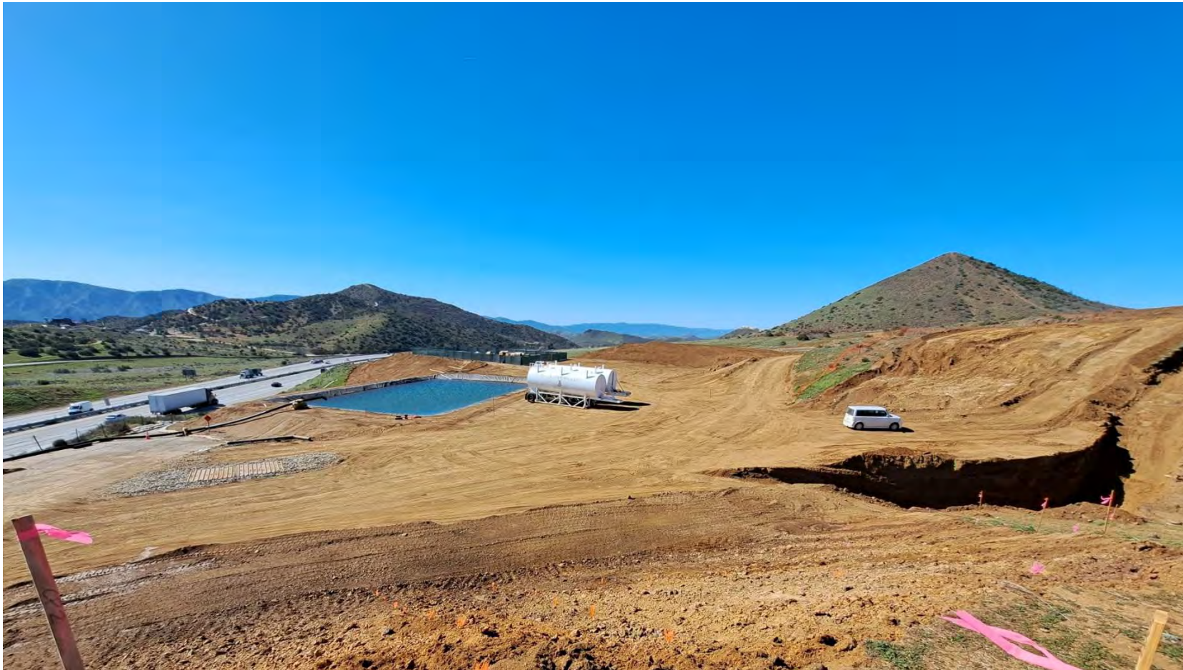
View from Valley Sage Road entrance to phase 1 facing HWY 14
