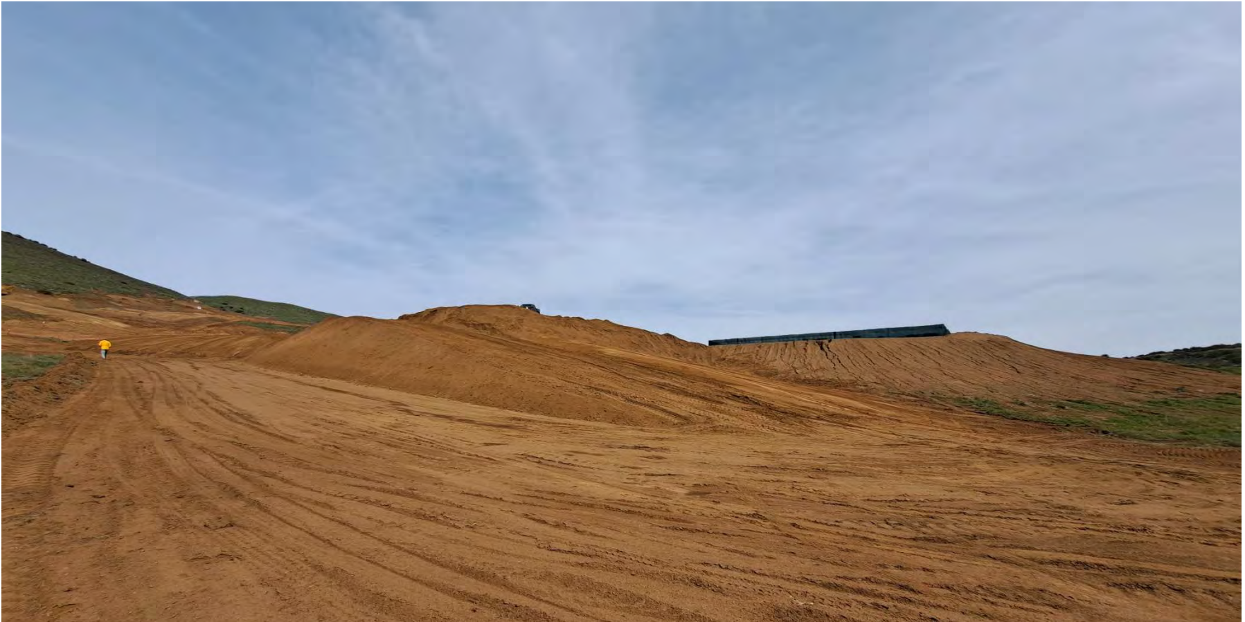
Picture of stockpile (of +/- 120000 CY of dirt) and construction equipment pad facing the graded area.
