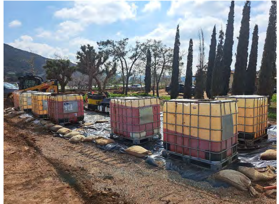
Reinstallation of BMP to ensure double containment around fuel tots.. (WM-4)
