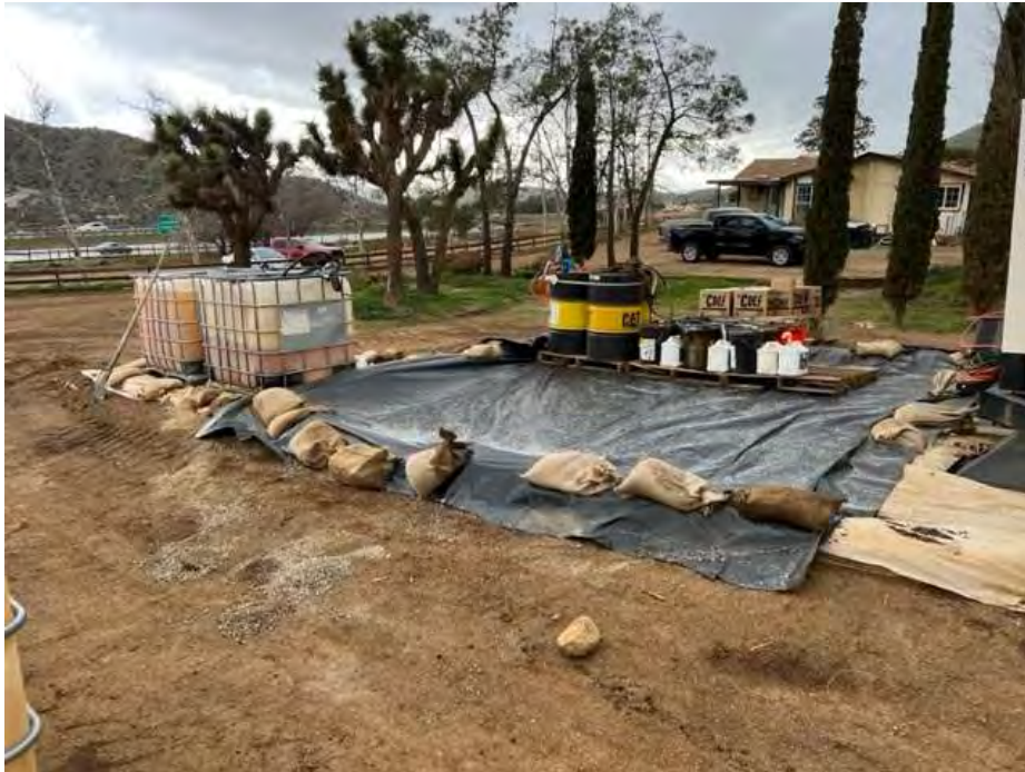
Reinstallation of BMP to ensure double containment around fuel tots.. (WM-4)
