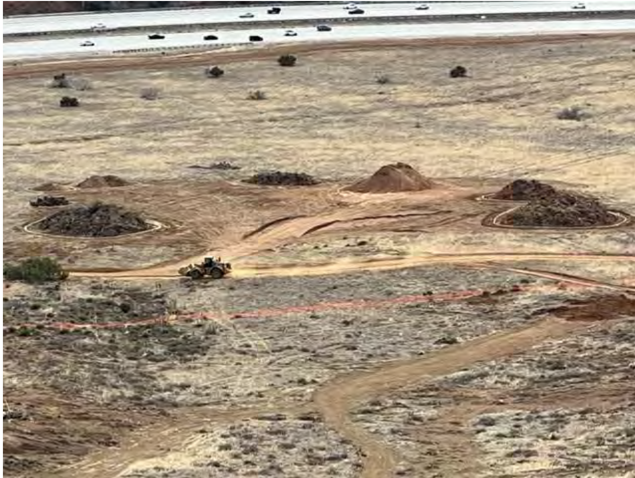
SWPPP installed in site spoils area ( BMP WM-8 )
