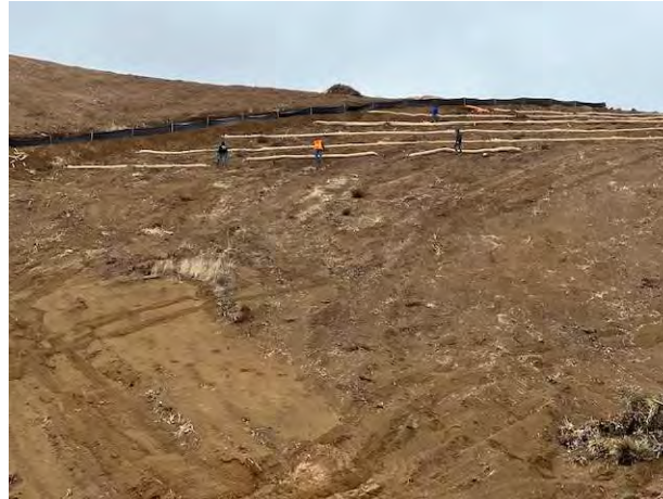
Straw waddle installation see Fig 1
