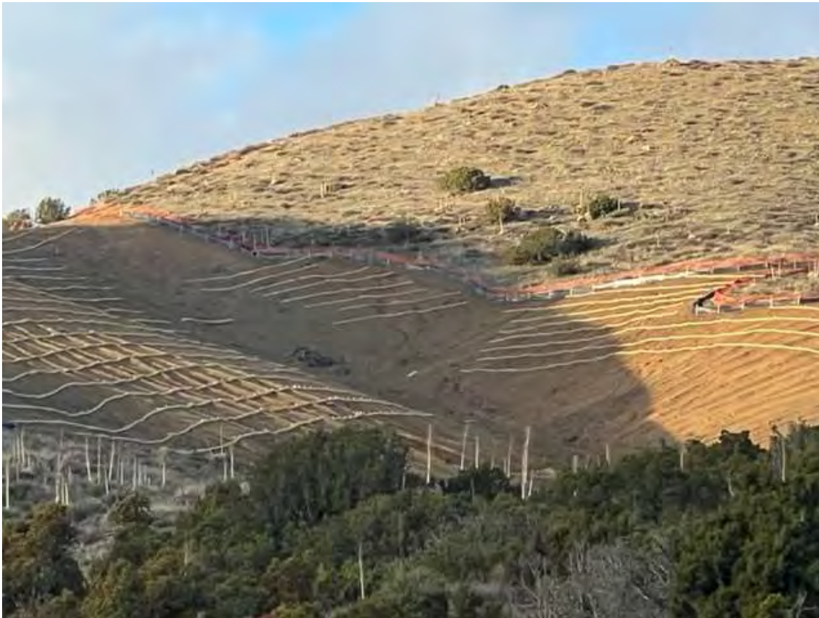
Installed soil erosion control as per approved winterization plan.
