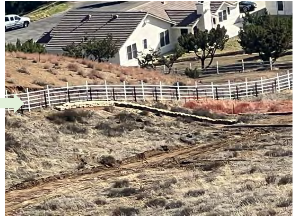
SWPPP Installed as per approved winterization plan, using sandbags on the eastern end of the property close to Mr. Estes's residence
