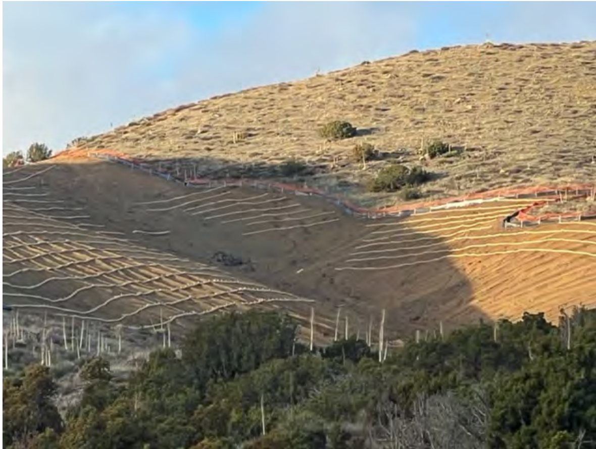
Installed soil erosion control as per approved winterization plan. see Fig 2
