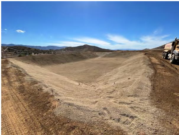
Pictures showing construction of pond, (lining pond with sand to ready it for the poly vinal liner) and tank pad for 12000gal elevated tanks.
