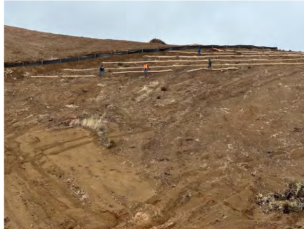
Straw waddle installation see Fig 1
