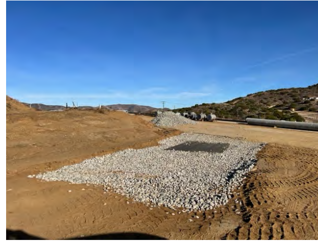
1. Track off system construction at phase 1 main entrance installed with 3" minus rock, fabric and grizzly plate
