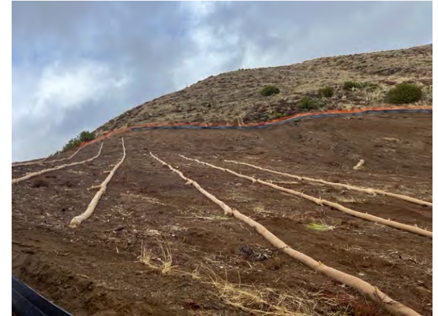
Straw waddle installation see Fig 1
