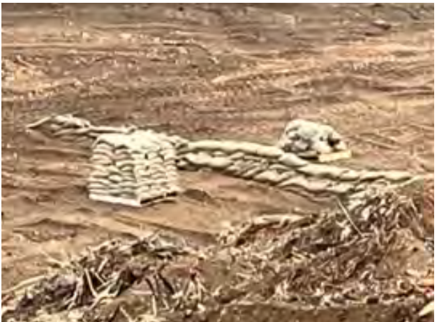
Dams installed in riparian area. see Fig 1
