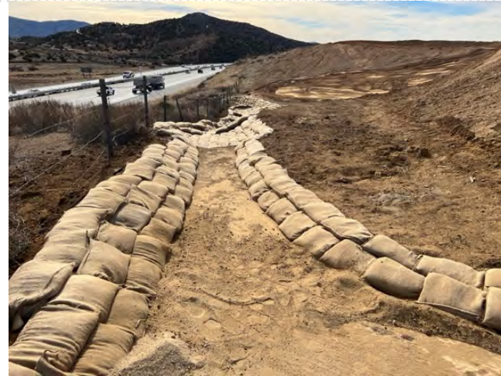
Sandbags used to line disturbed drainage area below the pond and close to the main entrance. see Fig 1
