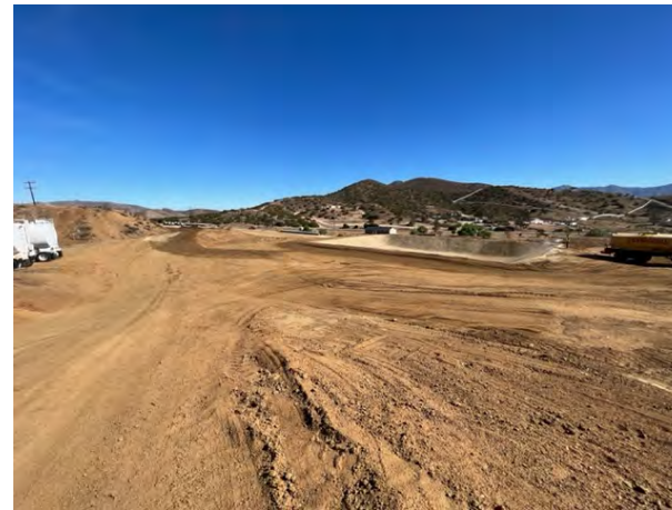
Pictures showing construction of pond, (lining pond with sand to ready it for the poly vinal liner) and tank pad for 12000gal elevated tanks.
