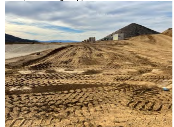
3. Preparation for water truck loading area
