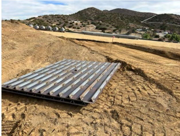
1. Track off system construction at phase 1 main entrance installed with 3" minus rock, fabric and grizzly plate
