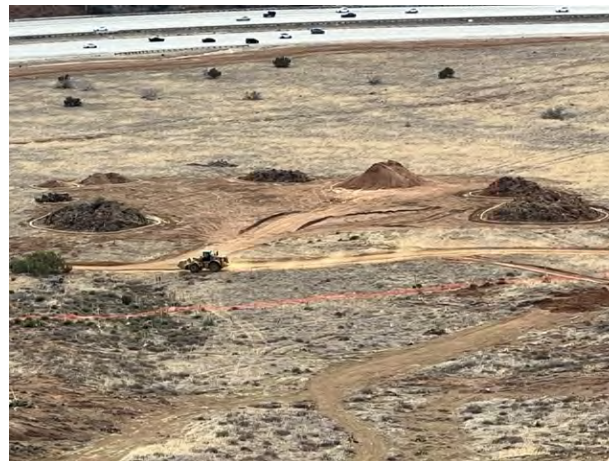
SWPPP installed in site spoils area and waddles installed around junk pile (WM-5) see Fig 1
