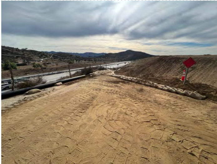
Sandbags used to line disturbed drainage area below the pond and close to the main entrance. see Fig 1
