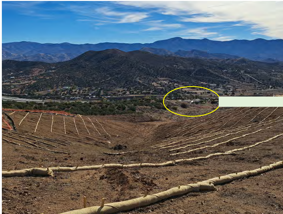
SWPPP Installed as per approved winterization plan, using sandbags on the eastern end of the property close to Mr. Estes's residence
