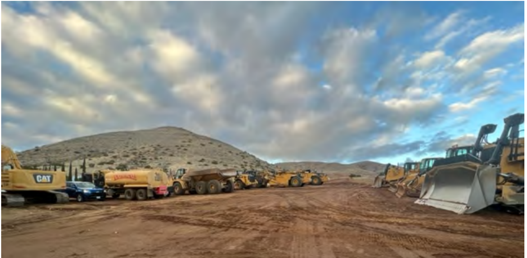
Heavy Equipment being used on site.
