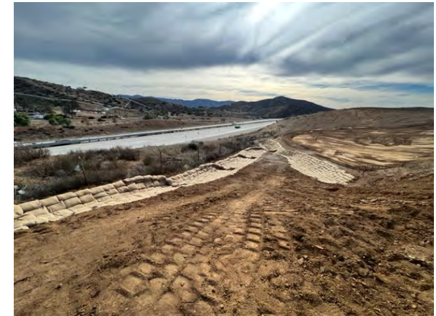
Pictures showing construction of pond, (lining pond with sand to ready it for the poly vinal liner) and tank pad for 12000gal elevated tanks.
