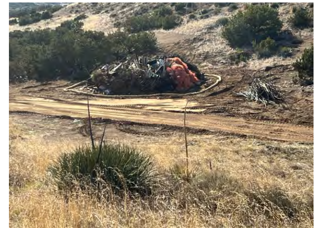
SWPPP installed in site spoils area and waddles installed around junk pile (WM-5) see Fig 1
