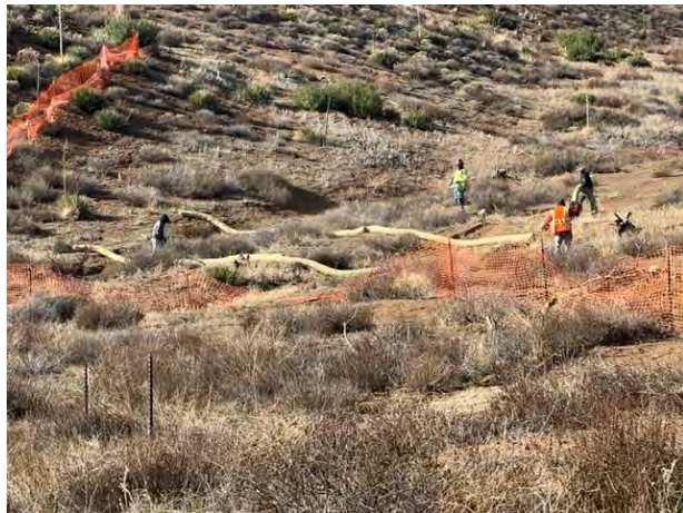
6 waddles installed in lower riparian areas. see Fig 1
